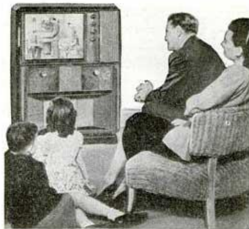
† Image is reflected by mirrors to a screen almost as large as a newspaper page in the RCA Victor console
