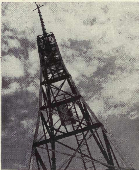
FIG. 19.—WABD antenna and tower at 515 Madison Ave., New York City. Crossarms on antenna is the video (picture) portion of the antenna and the donut on top is the audio (sound) portion of the antenna. ( Allen B. DuMont Laboratories, Inc. )
