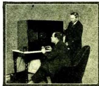
The receiver of Mr. Baird's television system, which is used with great success, it is stated.
