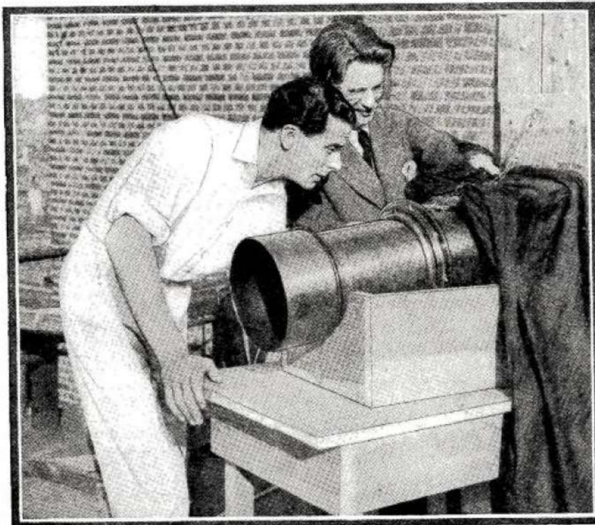
Mr. Baird (right) showing his television camera to an old schoolmate, Jack Buchanan, musical comedy star. Observe the light-gathering capacity of the lens, contained in the tube, behind which is the covered scanning mechanism.
