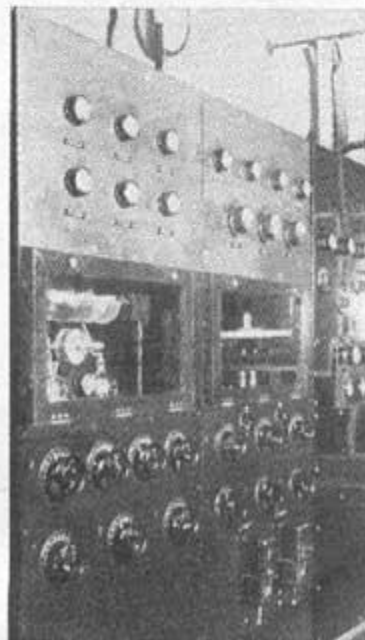
Transmitter panels of the Don Lee television station. They built them.
