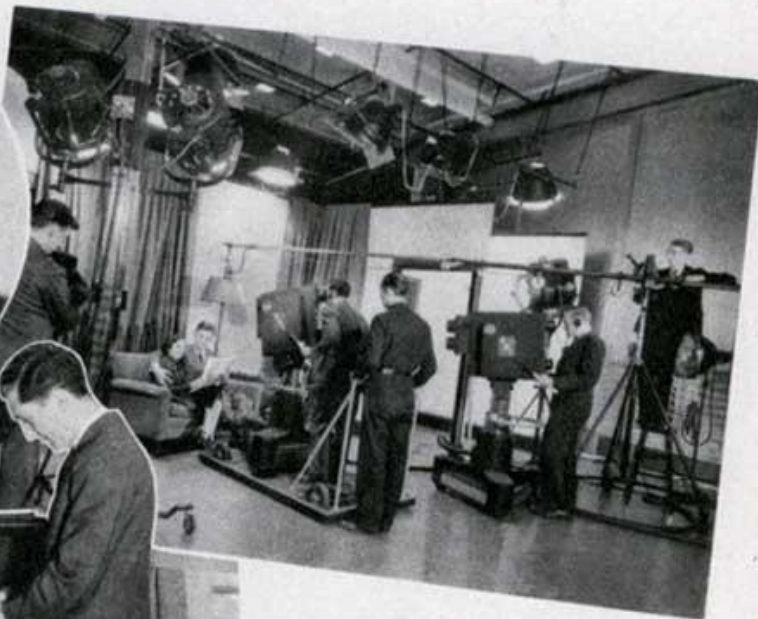
Television is photographed under the same conditions as a motion picture except that an Iconoscope camera is used. This scene is being photographed in the Radio City Television Studios. Left—A typical television set.
