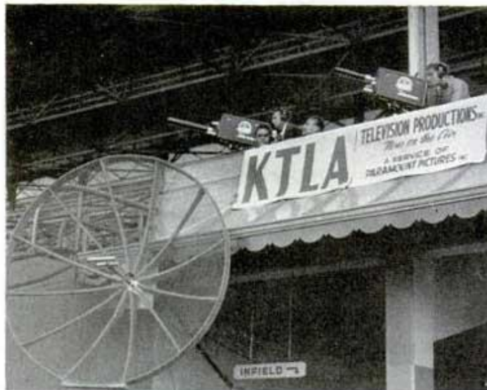
Line-of-sight "dish" antenna at baseball park beams pictures to main transmitter on mountain
