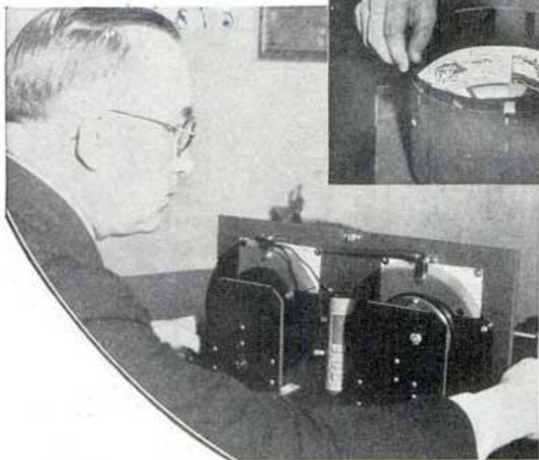
Two Views of Apparatus with Which Natural-Color Pictures May Be Transmitted and Received; the System Holds Great Possibilities for Television and Telegraphic Picture Service
