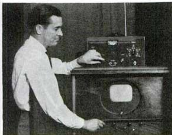
Miniature telecasting station (top cabinet) tests reception of receiving set below
