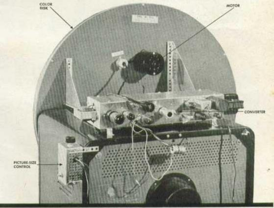
THESE PARTS ADD COLOR. The converter can be mounted either on top of the set as shown here, or vertically behind the cabinet, thus leaving the top entirely clear when the color disk is removed. This wheel unit, which rests on rubber feet and requires no fastening to your TV set, can be disconnected and quickly removed for black-and-white reception.
