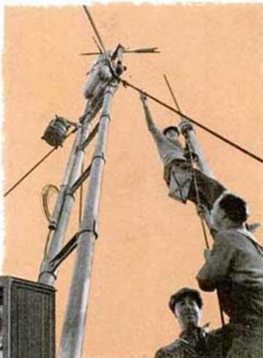
Workmen installing a lightning arrester to protect the antennas of a television station in the Empire State Building, New York City. Left, a modern television receiver with sight and sound circuits housed in a single cabinet
