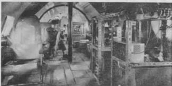
The engineer is orienting one of the directional antennas installed on the plane. Receiving equipment is at the right.
