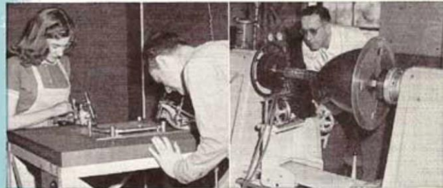
Color dot and aperture alignment requires use of high-powered magnifiers.
