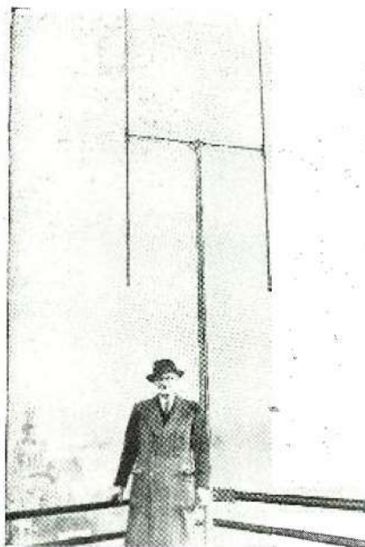
The British Televisors use this type of antenna for receiving.
