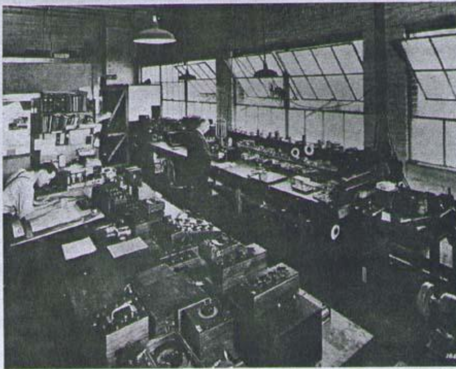
GILFILLAN ENGINEERING DEPARTMENT IN 1940
