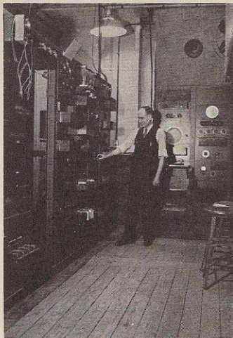
Television control room.
